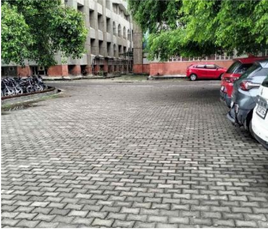
Paving stone installed in campus
